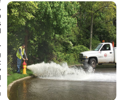
Municipal workers flush the water mains regularly
